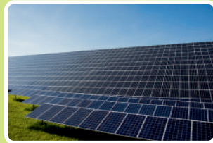
Solar Power Plant
