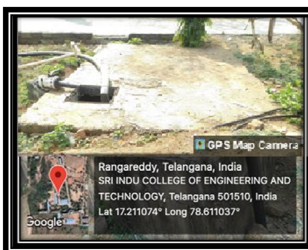
Waste Water stores in Tank and supplies through motor pump system
