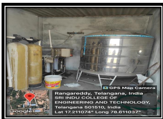
Recycling waste water through RO Plant
