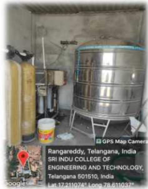
Recycling waste water through RO Plant
