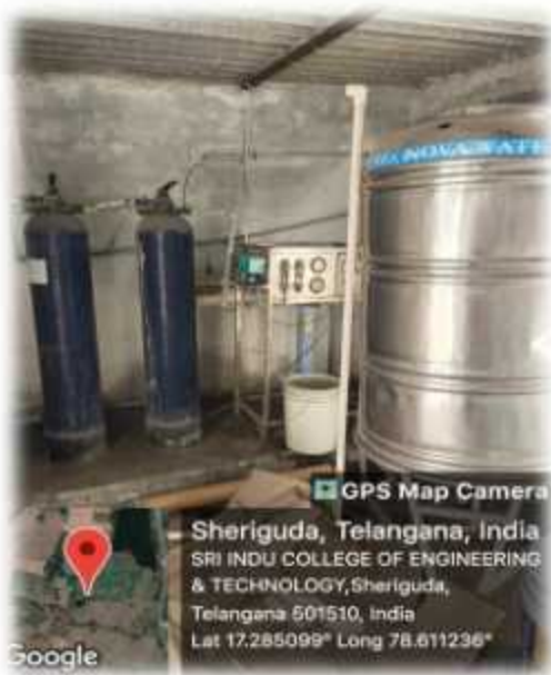
Recycling waste water through RO Plant
