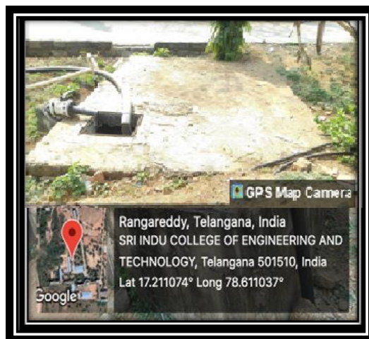
Treated Waste water stores in tank and supplies through motor pump system
